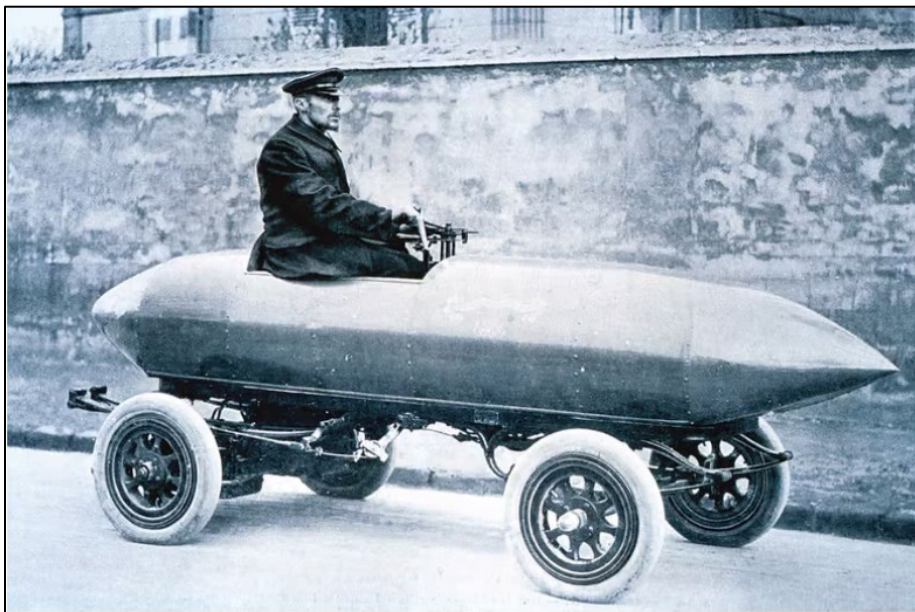
Jenatzy created the first "purpose built" car for a land speed record which he named the "Jamais Contente." The torpedo-shaped electric vehicle made extensive use of "partinium", a strong, lightweight and expensive alloy made of aluminum, copper, zinc, silicon and iron which had not been previously used in a car. The car ran 65.79 mph (105.26 km/h) for the final chapter in the duel.
